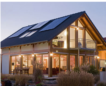
Off-grid power generation system
